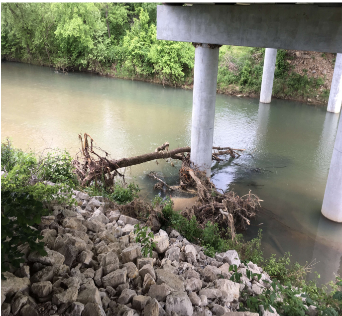
PHOTO 1 Description Drift accumulation on the right column of bent #2.
